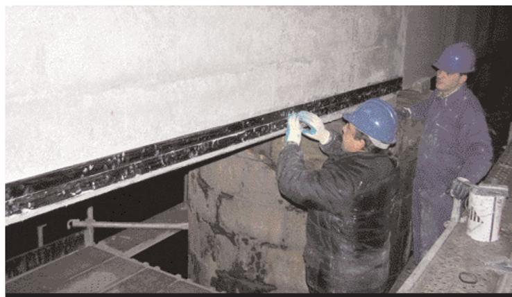
(TFC) of a width of 300 mm. In the places where the concrete was damaged, the steels were first passivated using epoxy resin agents. After that, we applied high-performance thixotropic mortar and acrylic paint to protect against carbonation. ■
