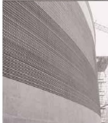
**The silo's capacity has been increased with the 117 additional prestressing that strengthen it over a height of 16 m.**
