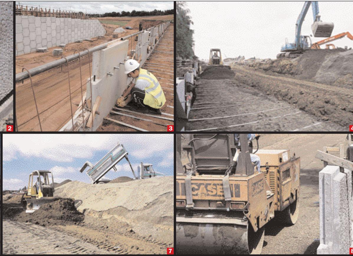
Prefabricated facing scales (1,3), metal or synthetic reinforcements (4,7), backfill material (4,6,7,8): the components of the technology place Reinforced Earth halfway between geotechnics and structures. After they have been laid, they form a composite material that is durable, effective and able to adapt to the most complex configurations.
