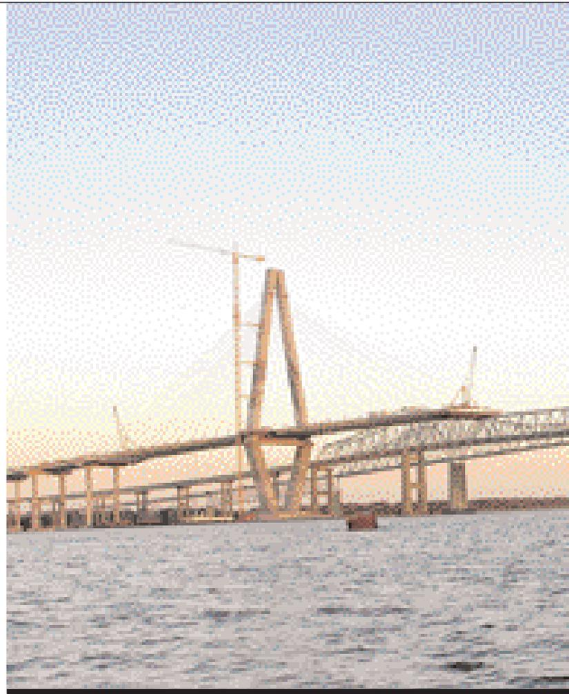
struction works, we had to erect "high-wind" stability cables to stabilise the structure when the average wind speed exceeded 75 km/h for an hour. Thanks to a system made up nails and a counterweight, the deck swung like a pendulum during the hurricanes.
