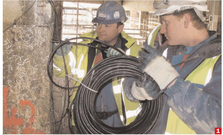
Once the titanium anode is installed, the installers make the electric connections.
