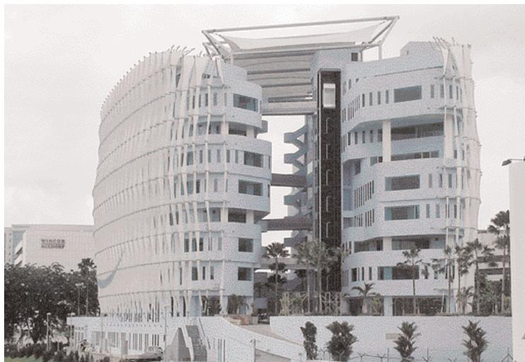
Freyssinet Singapore has taken part in designing and laying 23,711 m<sup>2</sup> of post-tensioned concrete floors for the headquarters of the computer services company Infineon Asia Pacific. The structure is made up of two oval-shaped buildings slightly out of line with each other, linked together by footbridges on the third, fifth, seventh and ninth floors.
