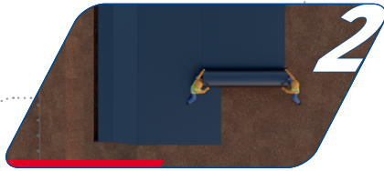
Non-woven geotextile installation for soil retention
