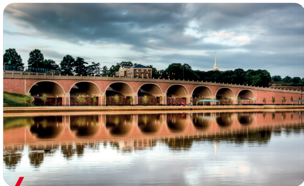
George Street Bridge, USA
