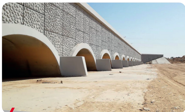
Wadi Stormwater Bridge, Saudi Arabia
