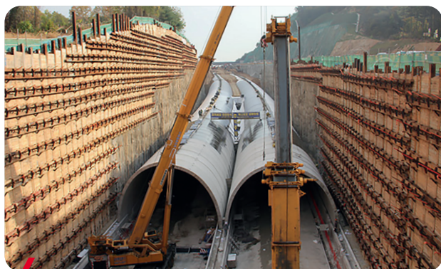
Suwon-Kwang Myeong Motorway (SKM) tunnel, South Korea
